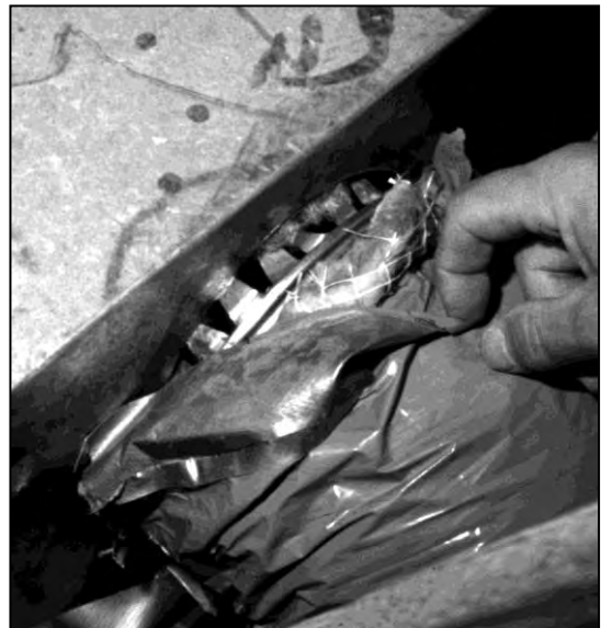
Supply Leak at Take-Off Connection
